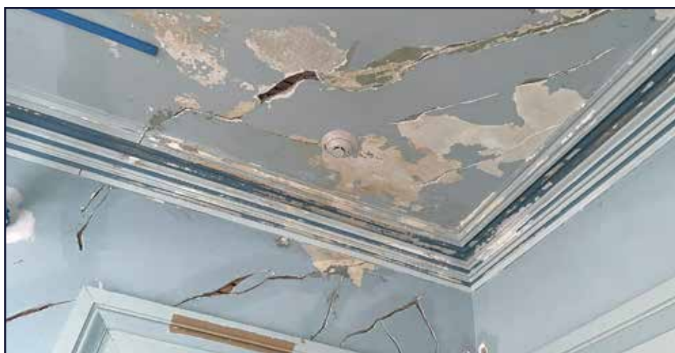
Walls and ceiling in SW storage room, 3rd floor, after damaged plaster was removed by FRHS volunteers and staff.
