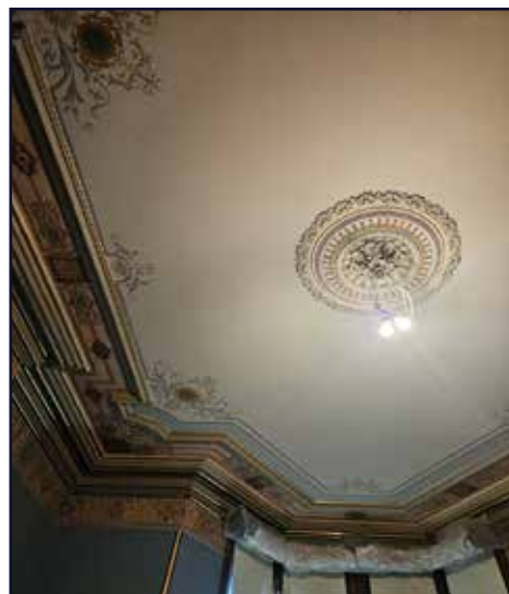
Left: Parlor ceiling showing repair to plaster from radiator leak. The radiator was replaced as part of the HVAC project. Right: Ceiling after restoration.
