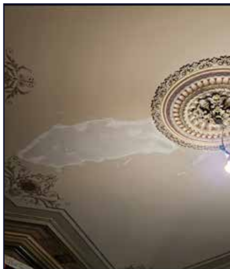
Left: Parlor ceiling showing repair to plaster from radiator leak. The radiator was replaced as part of the HVAC project. Right: Ceiling after restoration.
